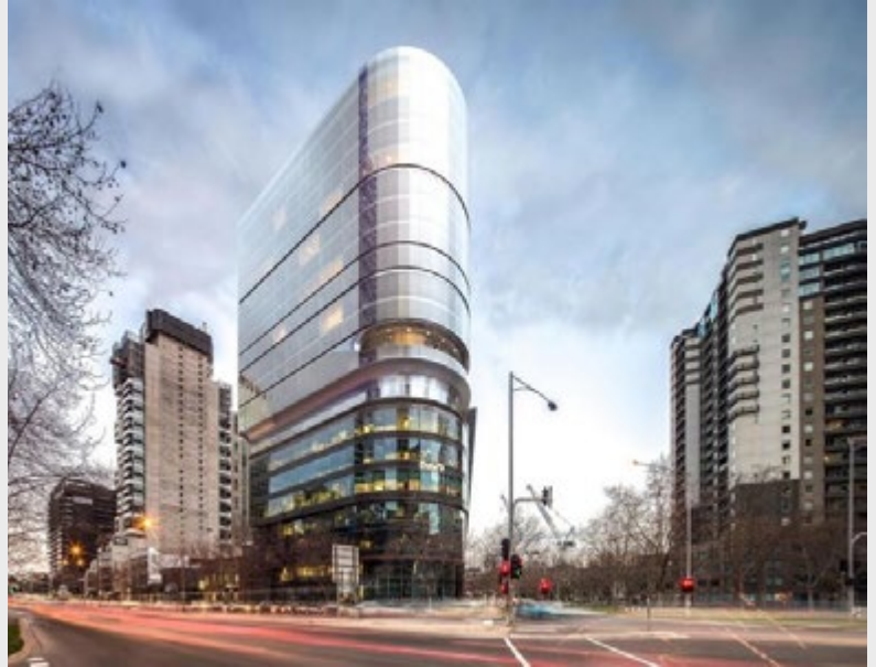
The world's tallest timber vertical extension, made possible by CLT
