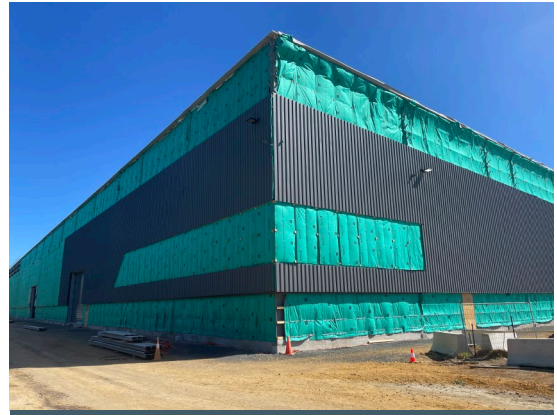
North-east corner of the NeXTimber manufacturing facility.
