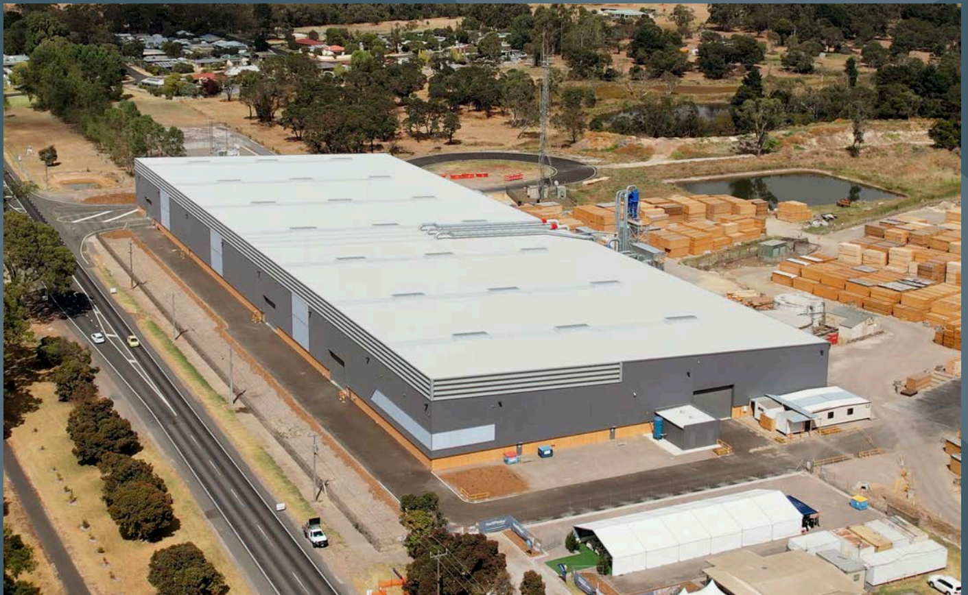
Timberlink's NeXTimber facility (pictured above) is Australia's only combined CLT and GLT (Cross Laminated and Glue Laminated Timber) radiata pine mass timber facility, and the first in Australia to be integrated with a structural timber manufacturing plant.
